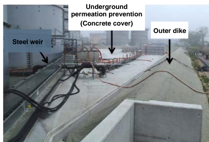
Figure 11 Situation of doubling dike and underground permeation prevention *2
