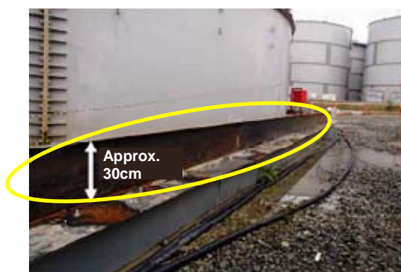
Figure 9 Situation of height raising of dike by steel plate *2 (H4 north area)
