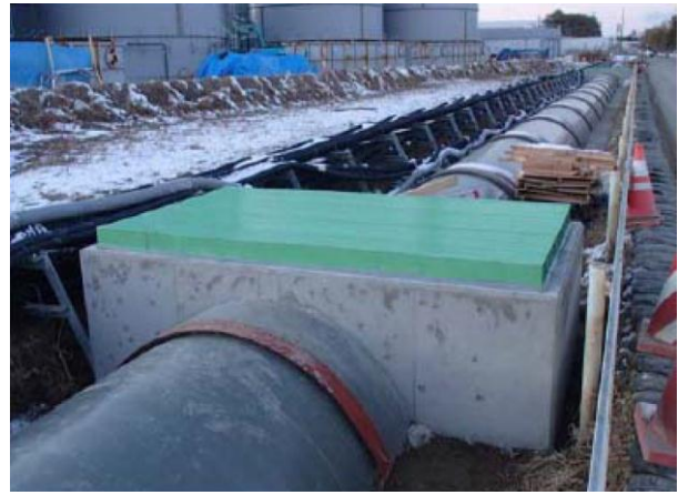
Figure 13 Situation of covering B drainage ditch *2
